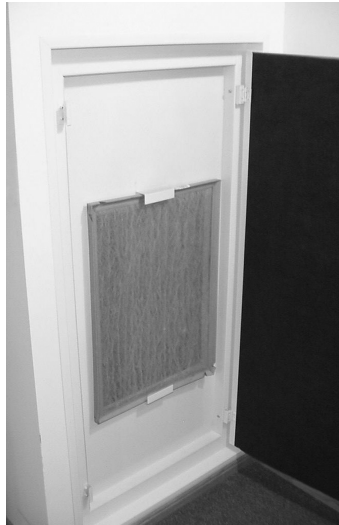
Figure 2. Return-air flush mounted hinged door
