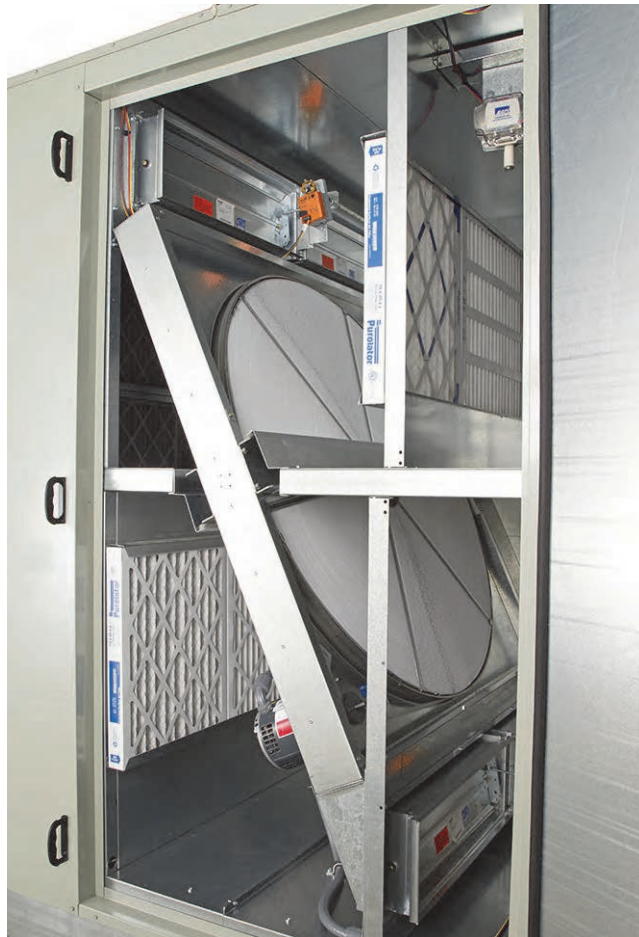
Figure 60. Total-energy wheel module
