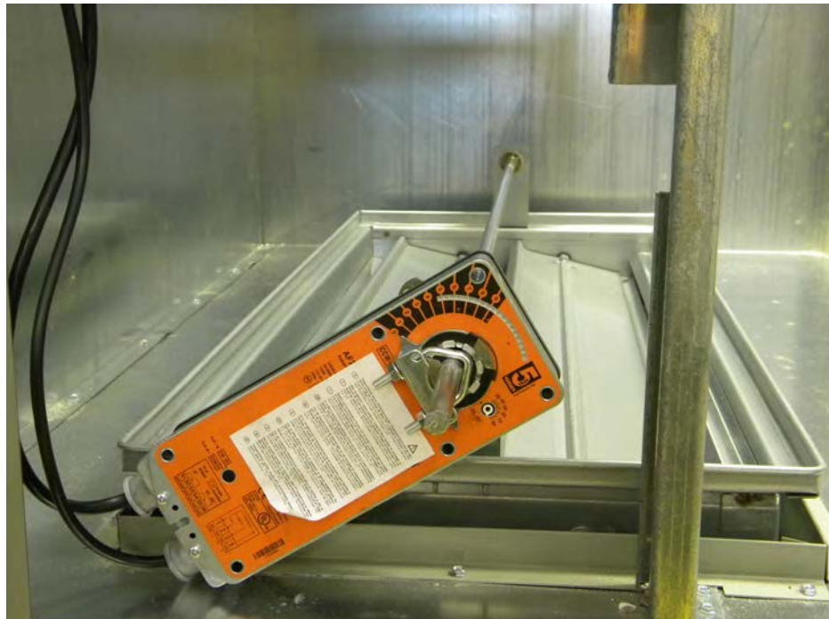
Figure 70. Return air damper
