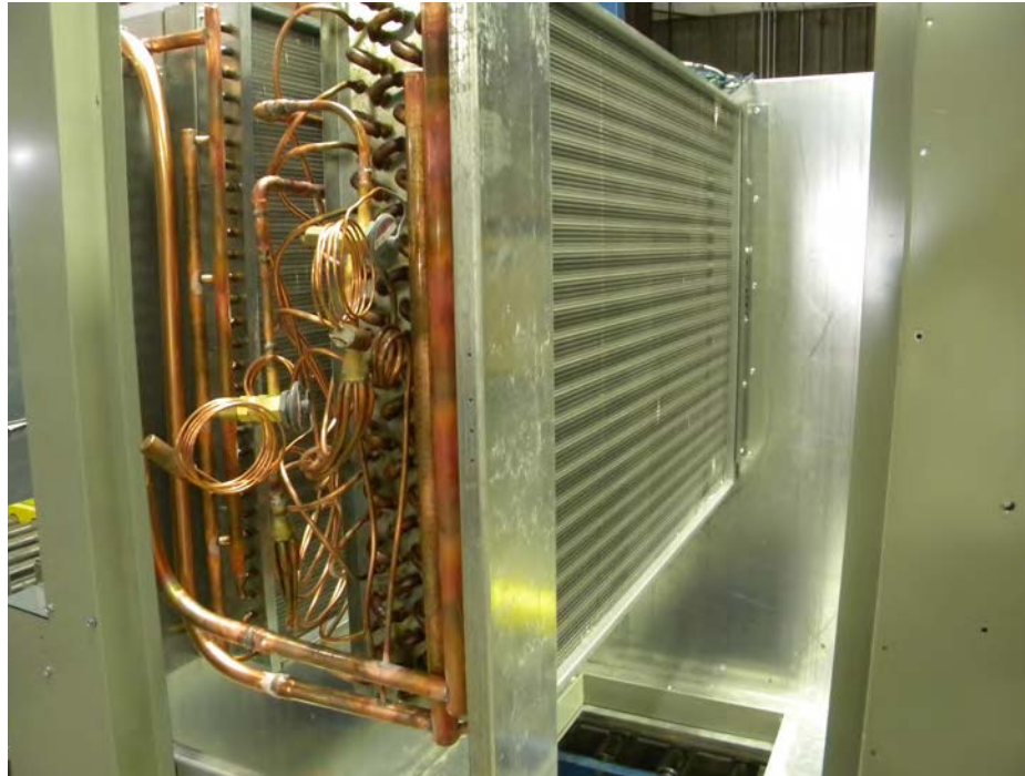
Figure 65. Evaporator and reheat coil
