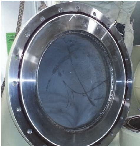
Figure 18. Installation of 1/8-in. GORE-TEX tape
