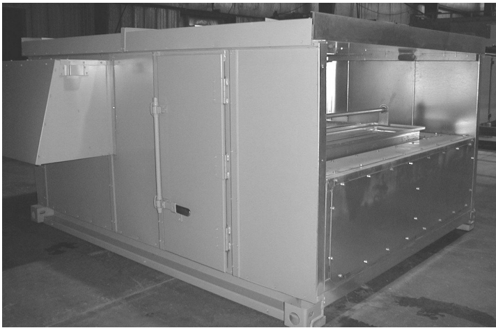
Figure 9. T-Series energy wheel section
