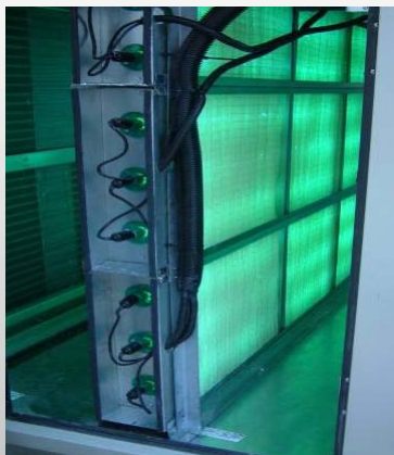
MERV 13 filter followed by Catalytic Air Cleaner (shown)
